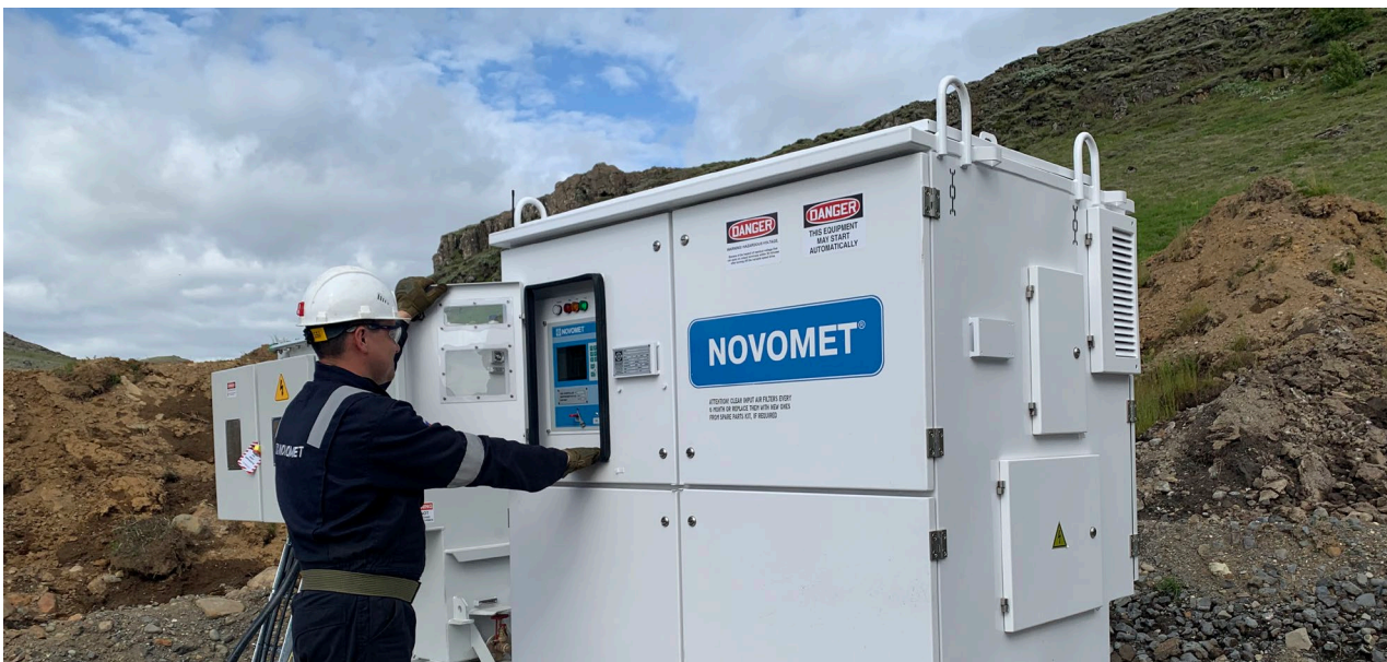
Geyser geothermal submersible pumps can be sped up, slowed down, and stopped as needed using a variable speed drive on the surface.
